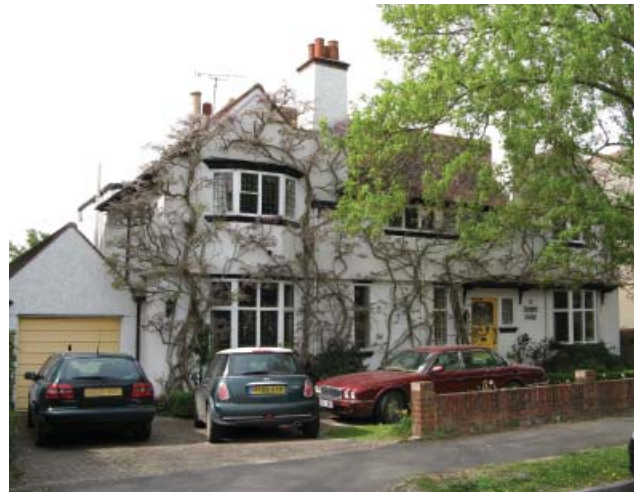
Inglefield Cottage, No.19 St Martin's Avenue
