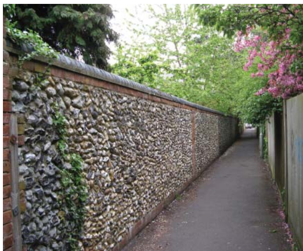
Flint cobble wall in alley between Rosebery Park and Worple Road
