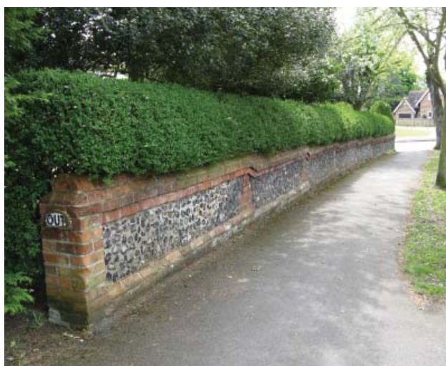
Flint wall outside No.2 St Martin's Avenue
