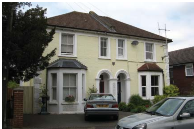
Protect buildings like these in Worple Road by an Article 4 Direction
