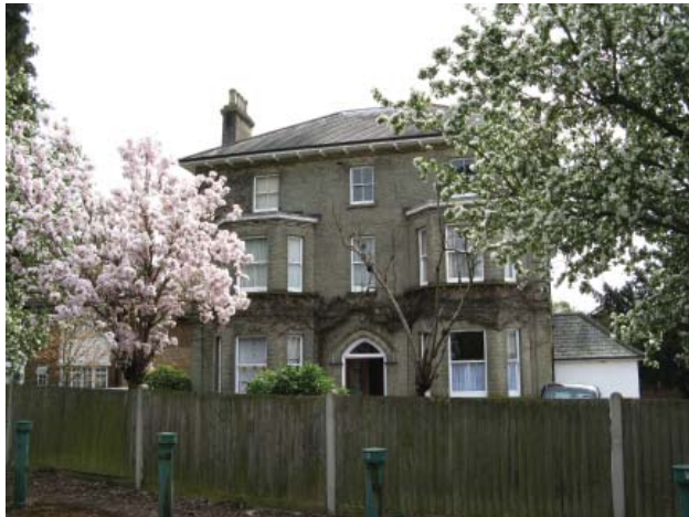
Sussex Court, Downside
