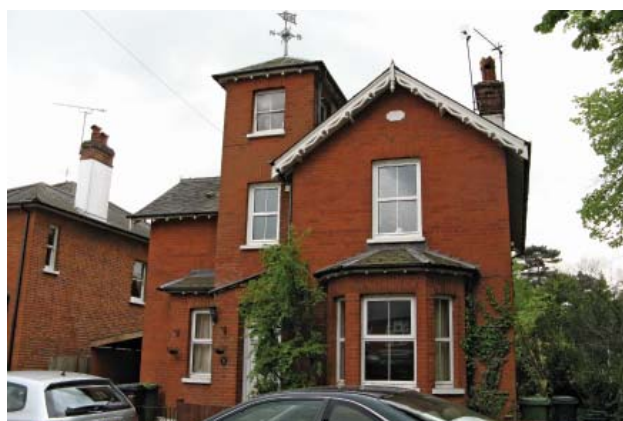
Turret Villa, No.3 Ladbroke Road
