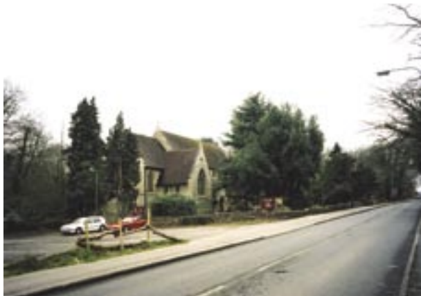
The flint wall around the church needs repairs
