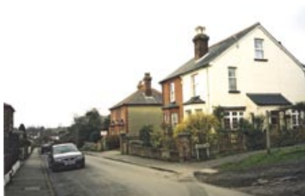
These houses in Lewins Road are “positive” buildings
