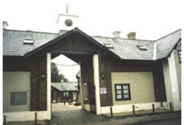
The former stables to Hookfield Hall, West Hill, have now been converted into houses
