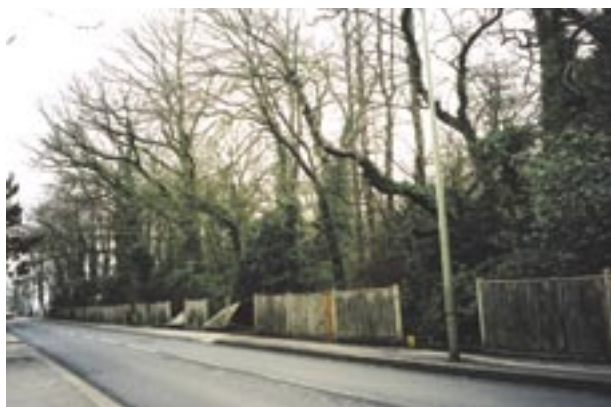
Damaged fencing on Christ Church Road
