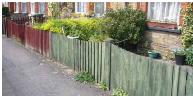
Low timber fences in Wyeth's Road
