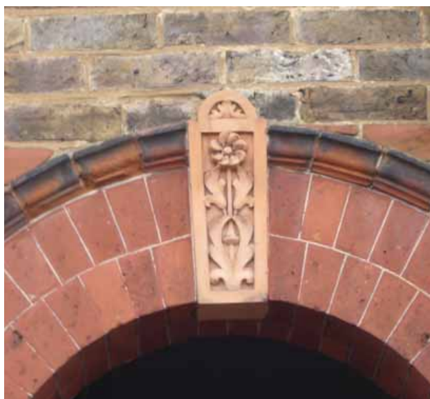
Brick and terracotta detail, Wyeth's Road
