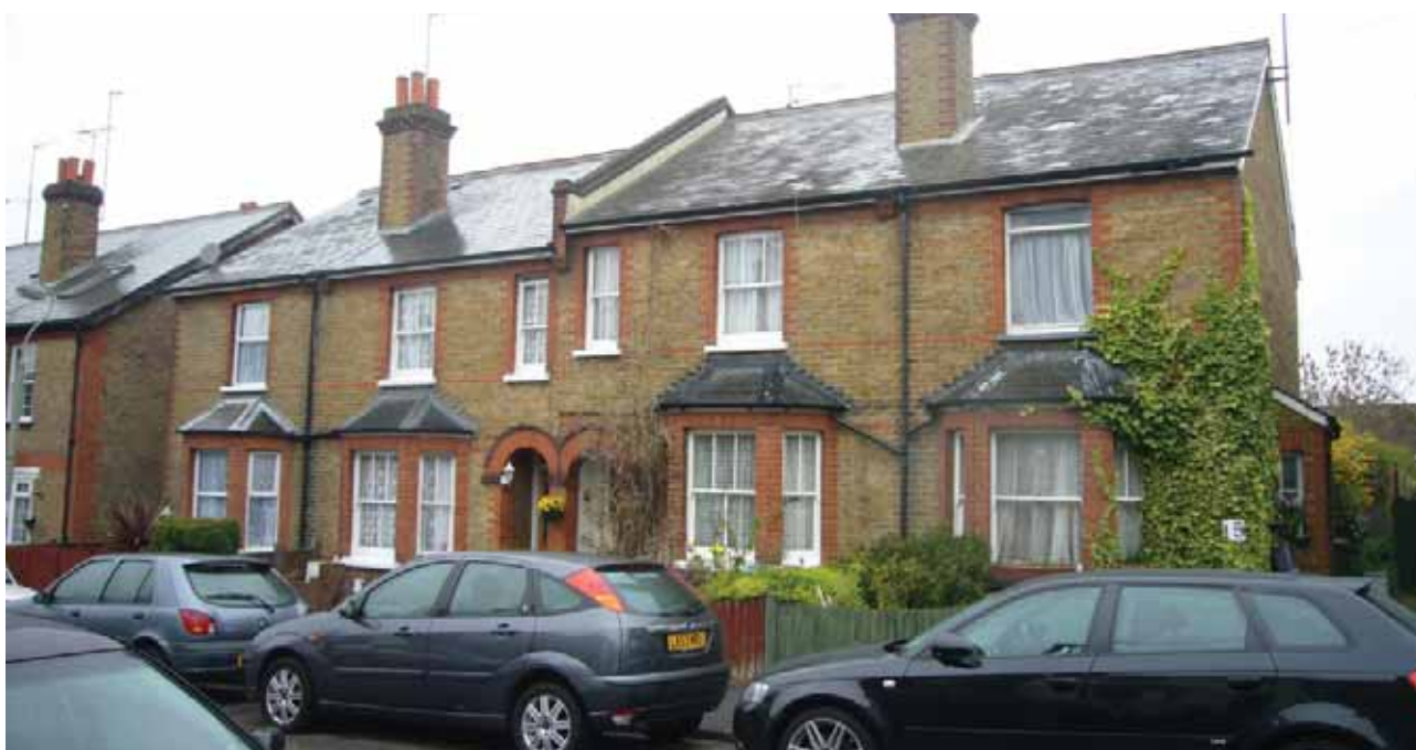
Nos. 33 and 35 Wyeth's Road
