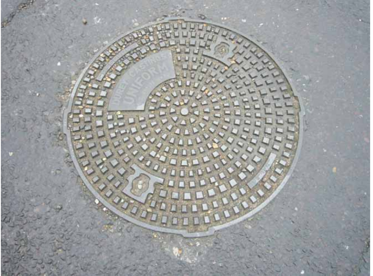
Manhole cover, Church Road
