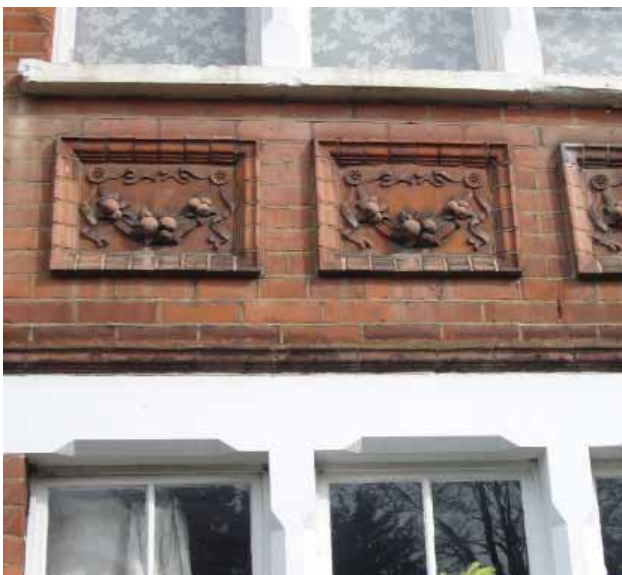
Decorative detail at no. 43 Church Road
