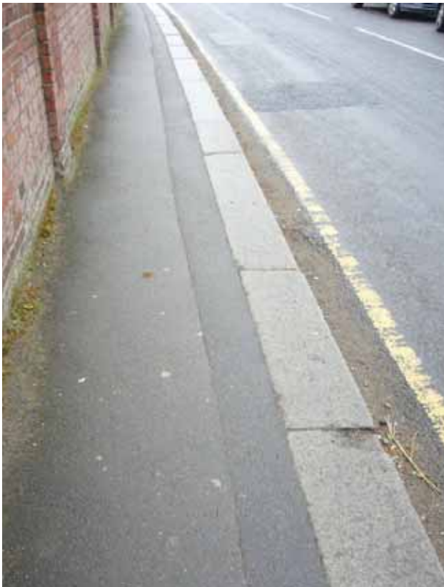
Natural stone kerb, Church Road
