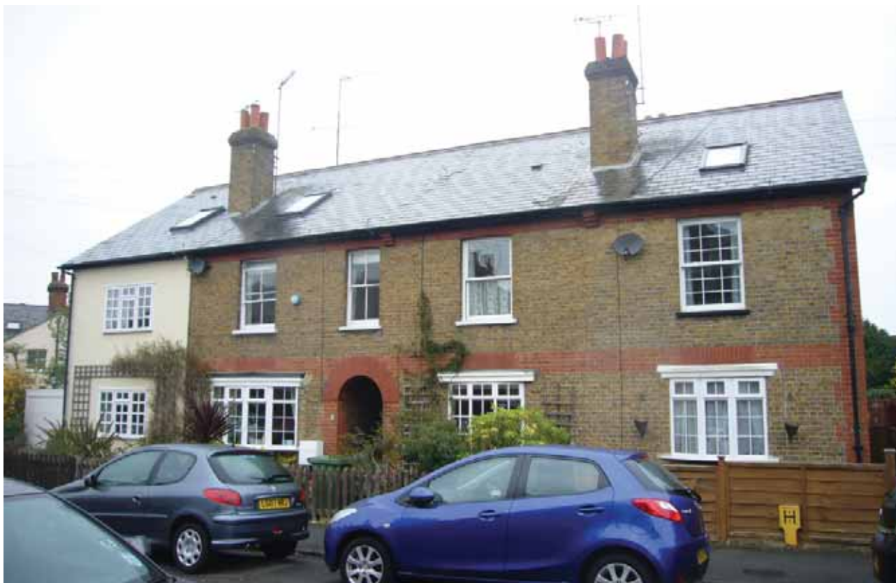
Windows have been altered in Wyeth's Road
