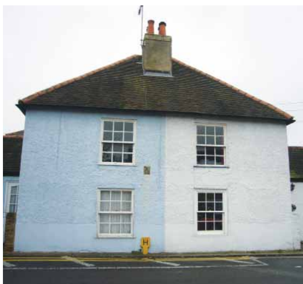
Nos. 1 and 3 Lintons Lane (grade II)
