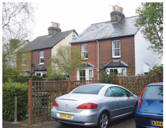
Car parking in Victoria Place
