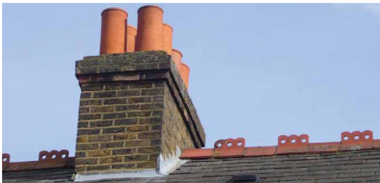
Typical brick chimney stack, clay pots and ridge tiles
