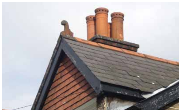
The conservation area has a lively roofscape (Middle Lane)
