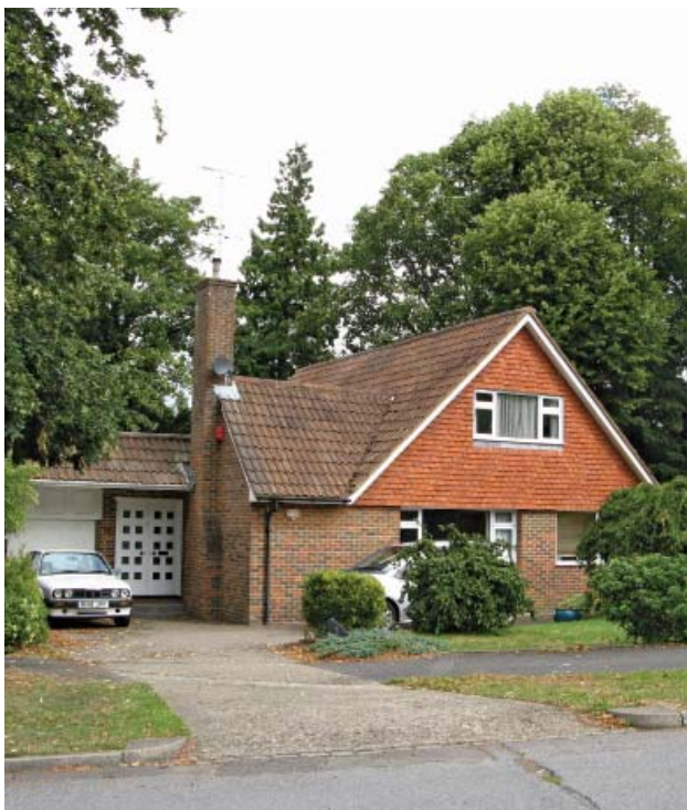
The house in The Ridings retains its original tile hanging and clay pantiles on the roof
