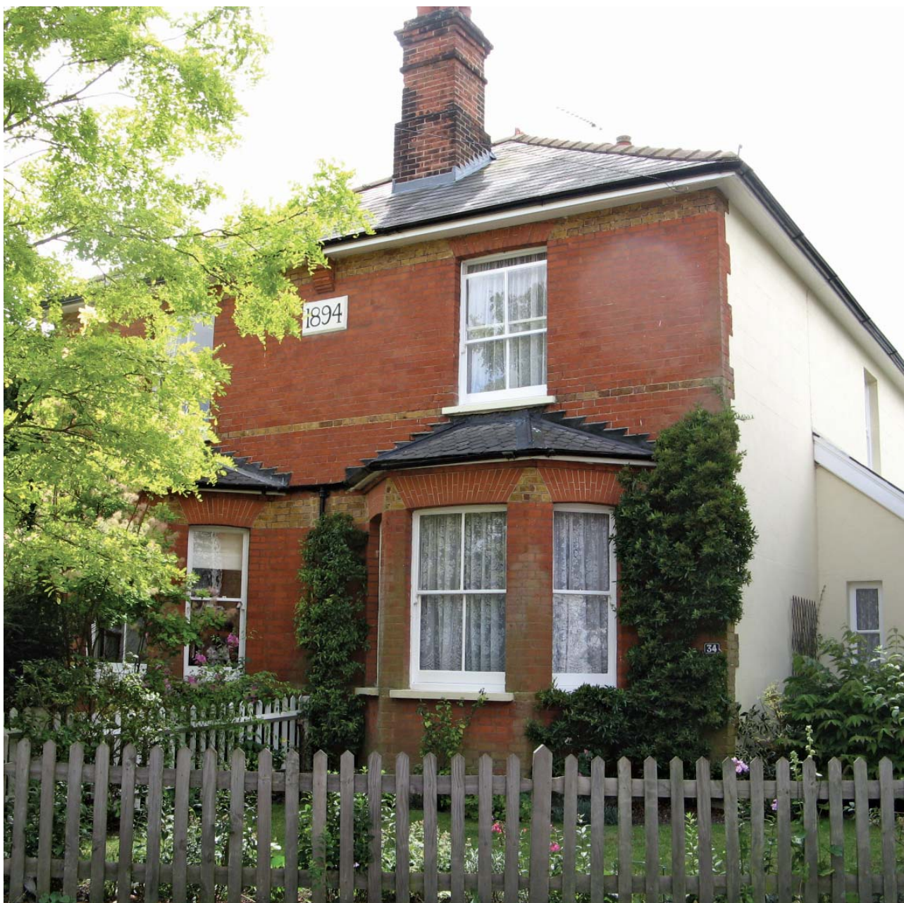
Traditional palisade fencing in front of No. 34 College Road
