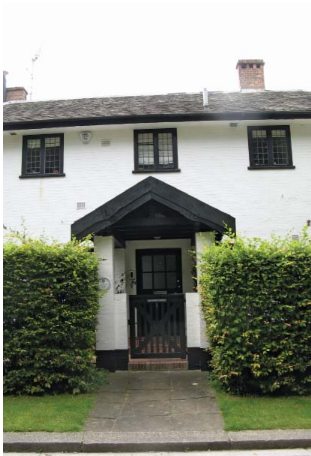
Bayfield House, No. 1 College Road
