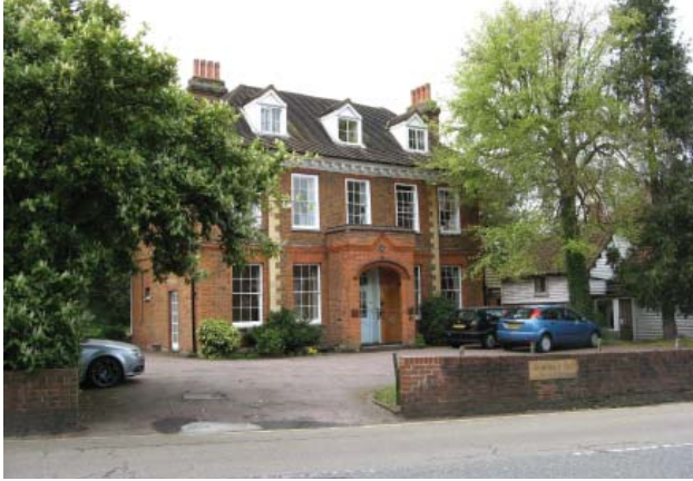
No.18 Church Street
