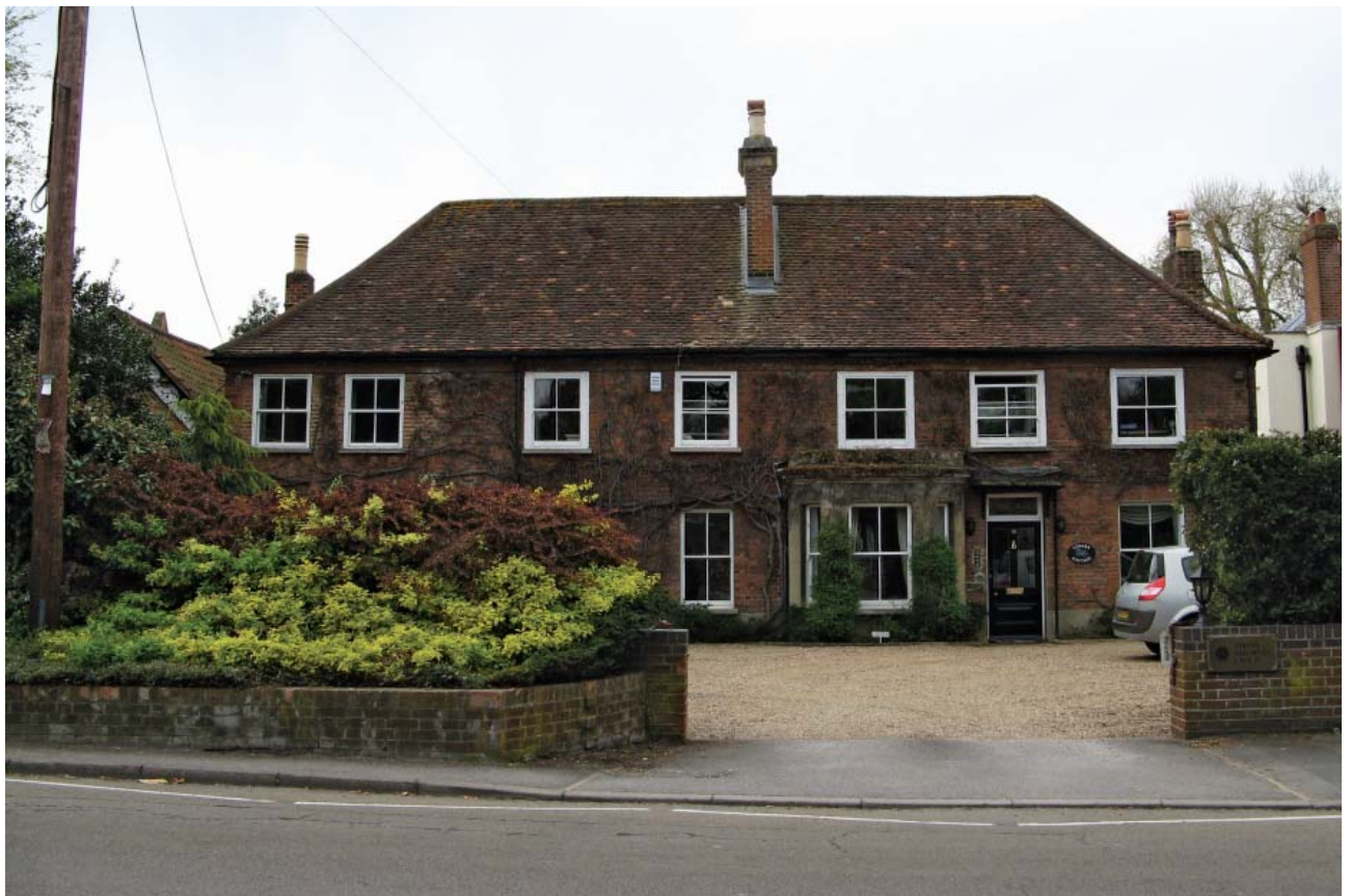
Handmade clay tiles on the roof of Cedars Cottage, No.16 Church Street
