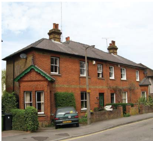
'Positive' historic buildings in Worple Road
