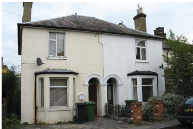
Satellite dish on Heathcote Road property
