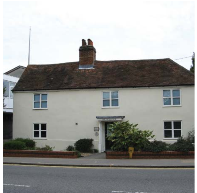
The Hermitage, Church Street
