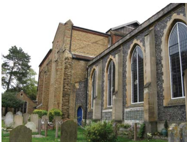
Greensand extension to St Martin's Church
