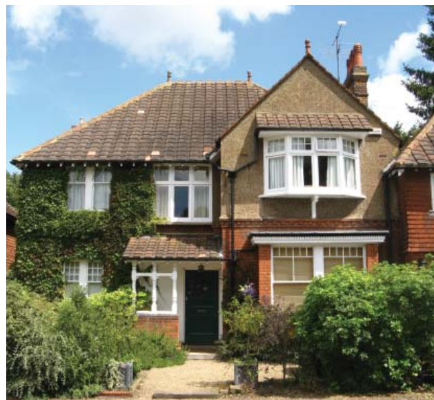
House in Lynwood Avenue with square inter-locking tiles
