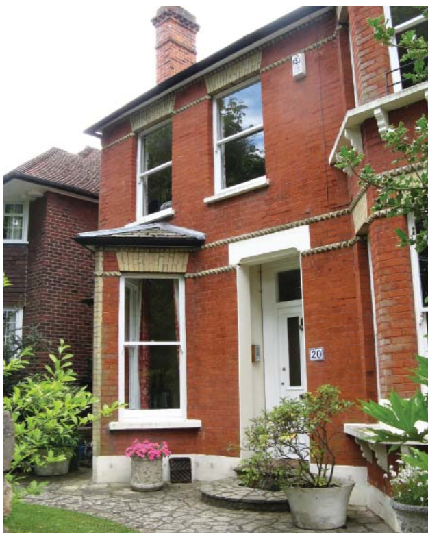
Detail of house in College Road
