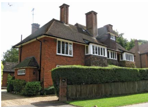
The Haining, Downs Avenue
