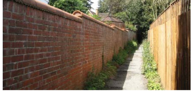
Brick wall in alley off Downs Avenue
