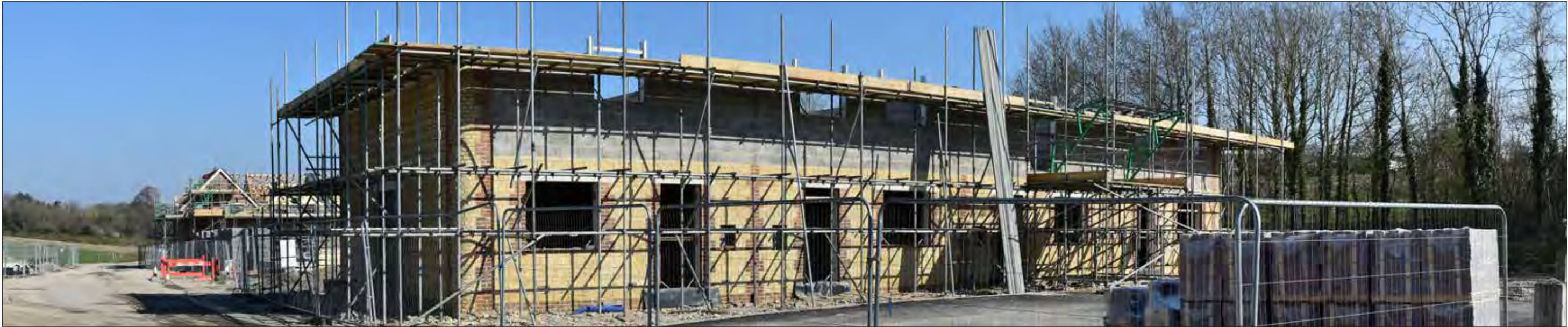
Photograph B View looking northwest from Bridleway 33, illustrating the on-going construction works of 20 new homes adjacent to the Site.
