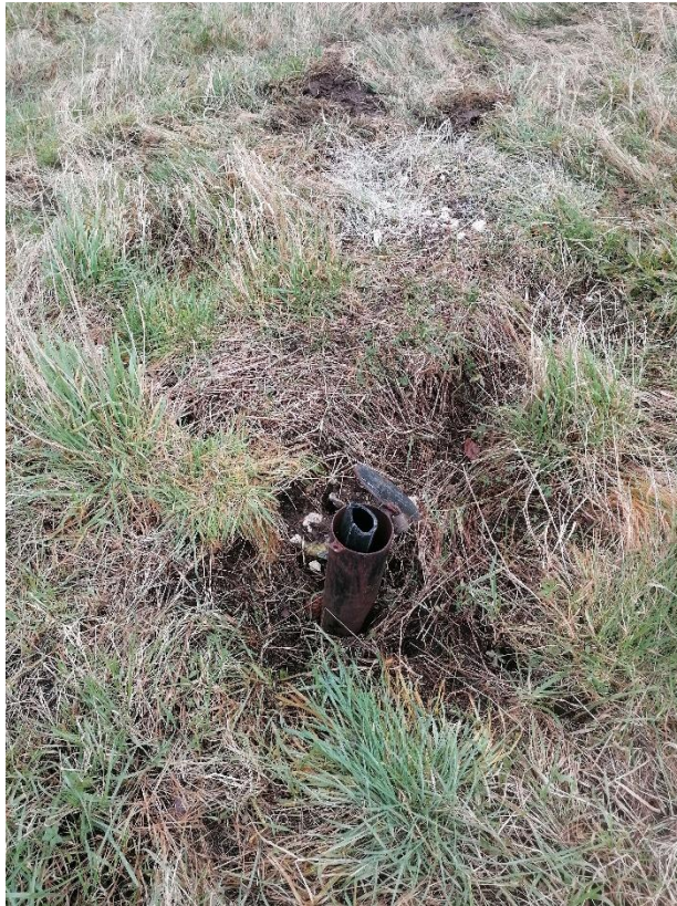
Damage borehole cover at north of Site
