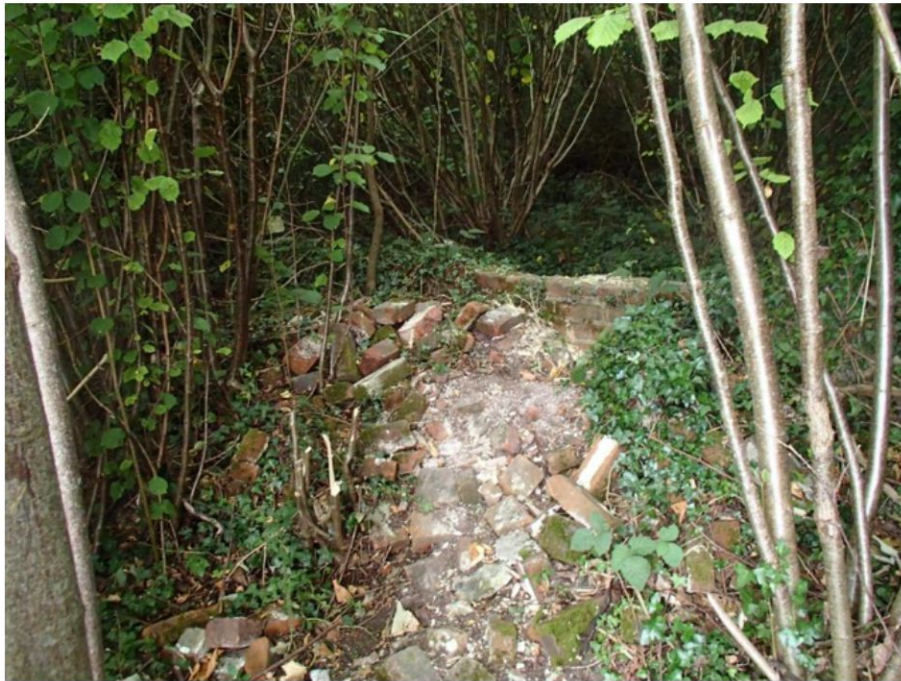
Plate 7.9: Wall collapse
