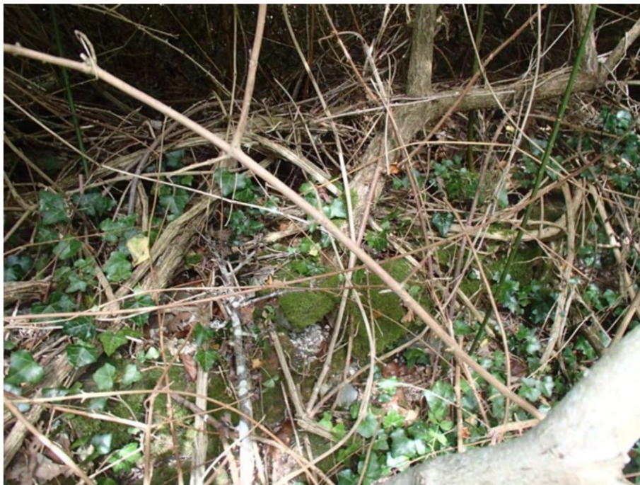
Plate 7.12: The state of preservation of the wall at the west end
