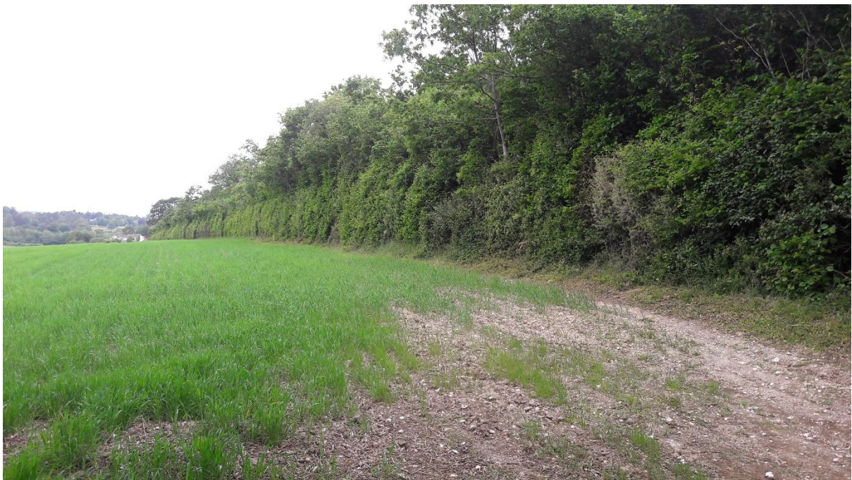
Plate 6: Dense scrub and trees along the external face of the south-west wall, facing north.
