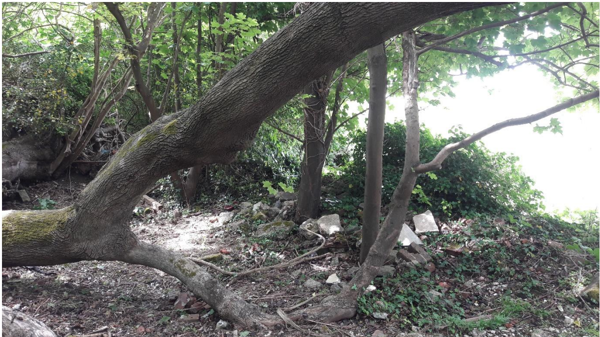
Plate 4: The remains of the west wall, facing south-west.
