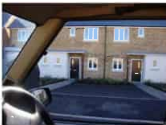
Ground sloping down from road towards low threshold properties in new St Ebbas development
