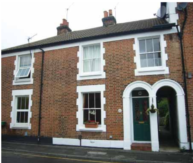
Red brick houses, Adelphi Road
