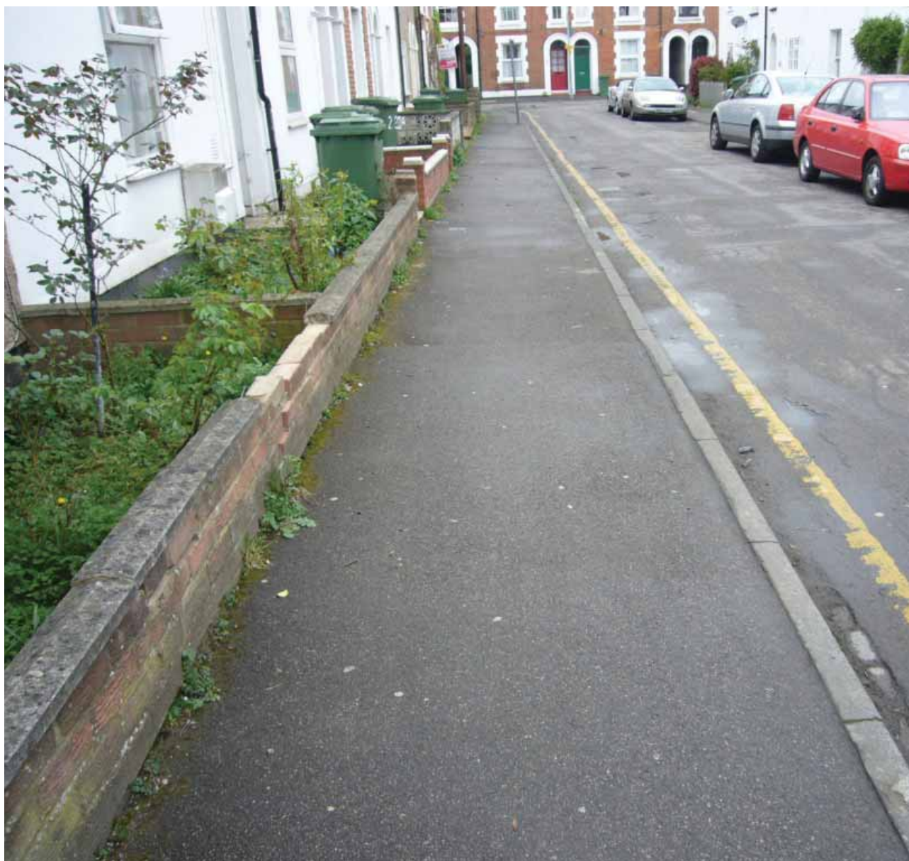
Front garden and boundary walls, Adelphi Road (south side)
