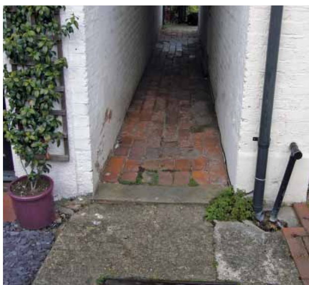
Brick pavers at nos. 1 and 3 Church Road
